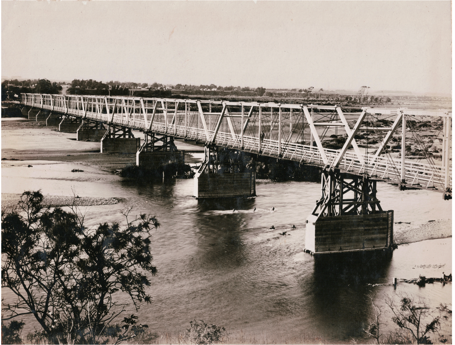
The first bridge at the end of Fitzherbert Avenue Palmerston North ,circa 1900
